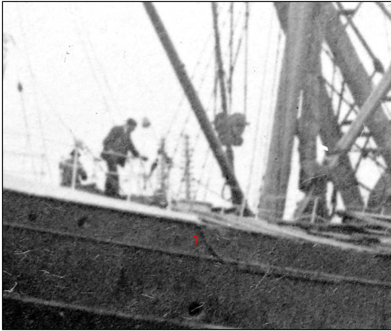
Figure 105: Details of scalloped foredeck bulwarks reduced around forward hatch 1 (1) (Image: After Green c 1900 (# gr005471) Nemesis at Wharf BW v SLV collection gr005471)
