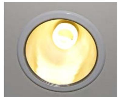
**Figure 19:** Compact fluorescent replacement lamp in recessed downlight
