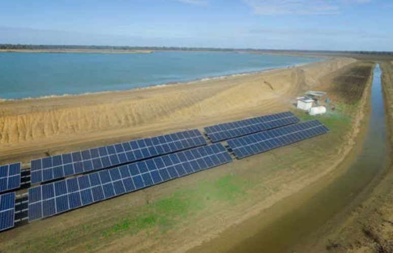
Solar-diesel hybrid powered irrigation system Photo: W Pratt/OEH
