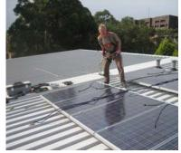
North Sydney College is the first of TAFE NSW Northern Sydney Institute's colleges to install a 1.980 kW solar grid interactive system. The panels can generate 8.3kWh of electricity a day. This translates to a 2.7 tonne reduction in greenhouse gas emissions.
