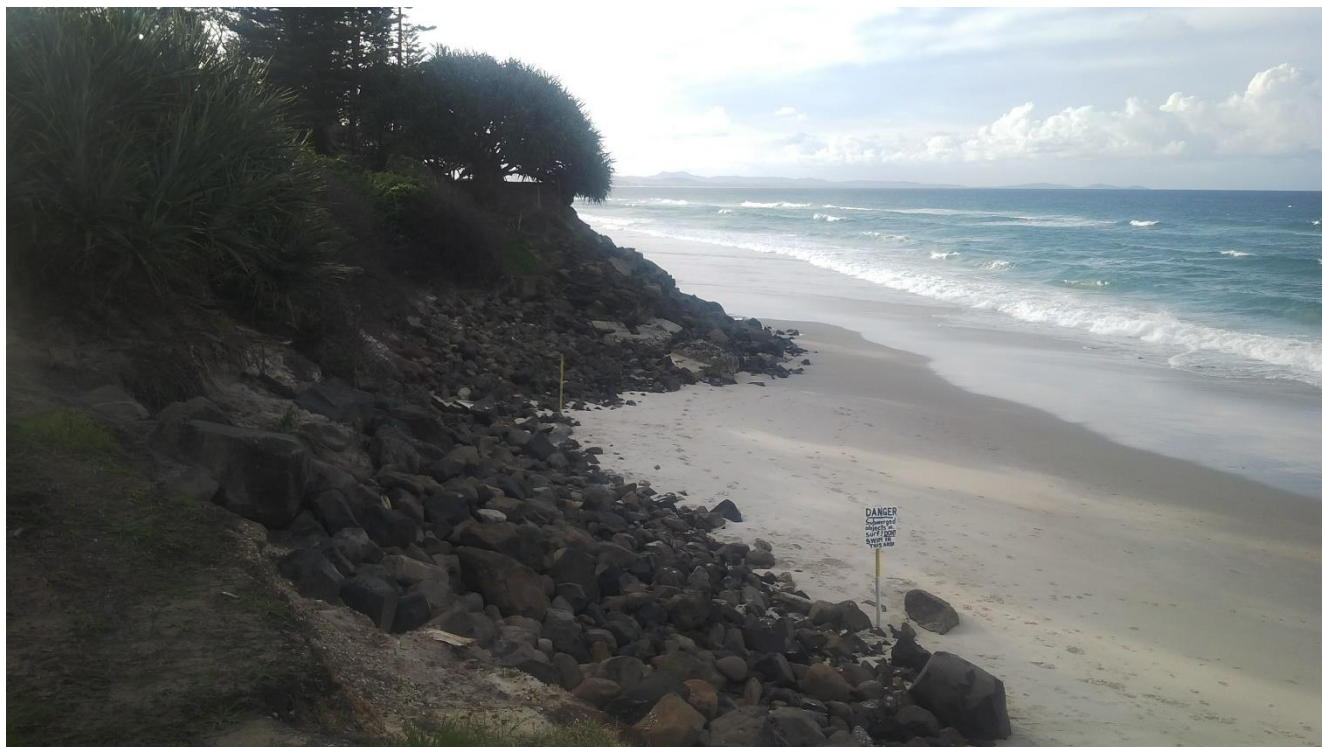
Figure 4 Toe and adjacent wall to southward exposed during erosion in 2013 (ICM photo)
