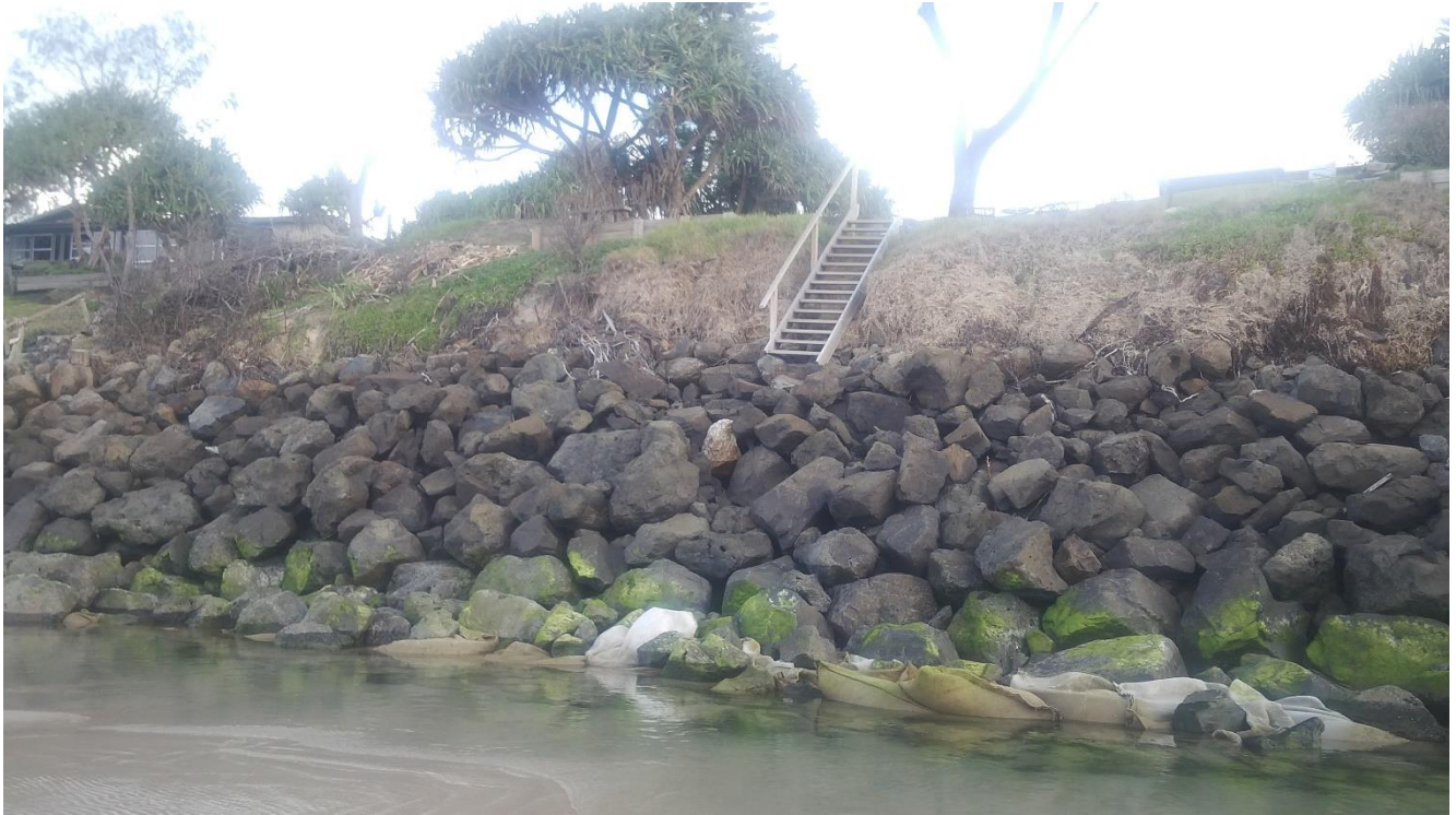
Figure 4 Toe and adjacent wall to southward exposed during erosion in 2013 (ICM photo)
