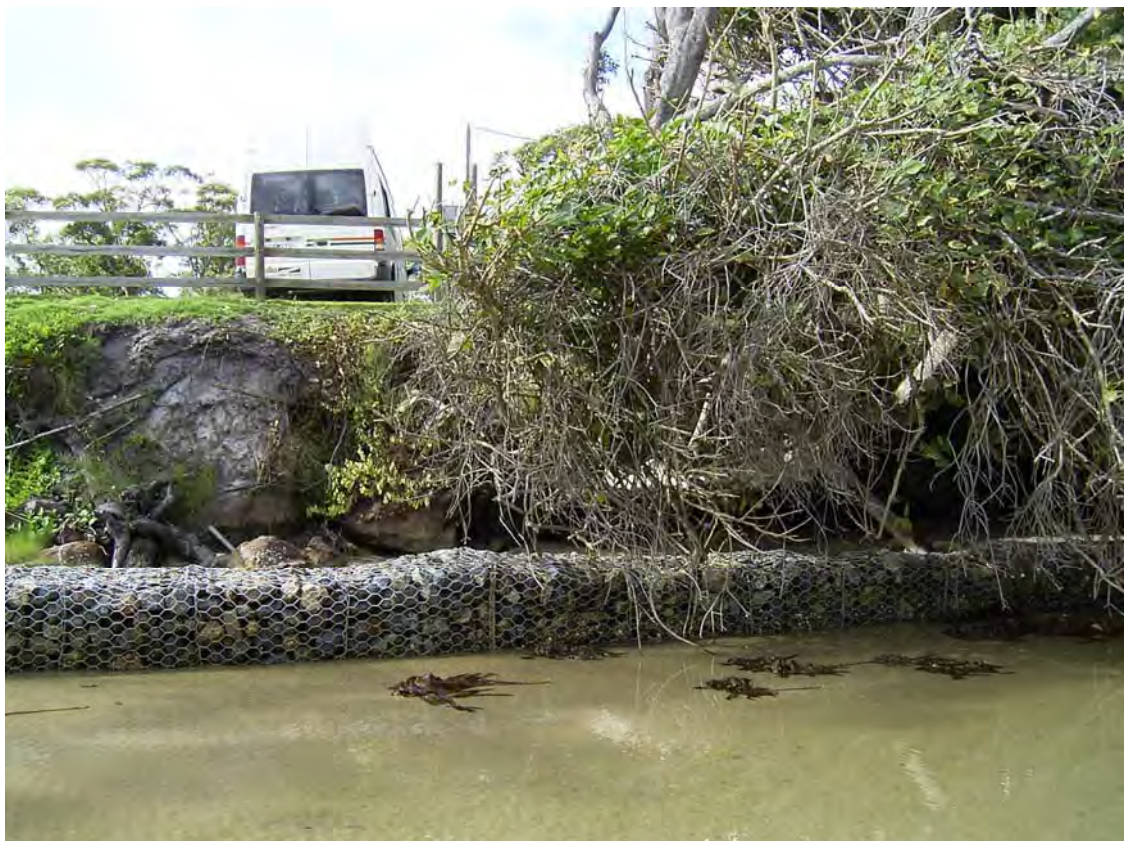
Photo 8 – Ch 185, Note scour and erosion to bank behind the gabion toe.
