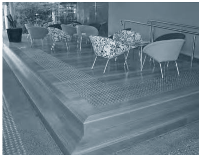
Hardwood floor made from recycled electricity poles
