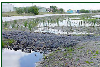
Rehabilitated stormwater drain
