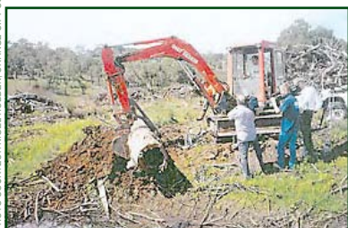
Placing a hollow timber log for fish habitat
