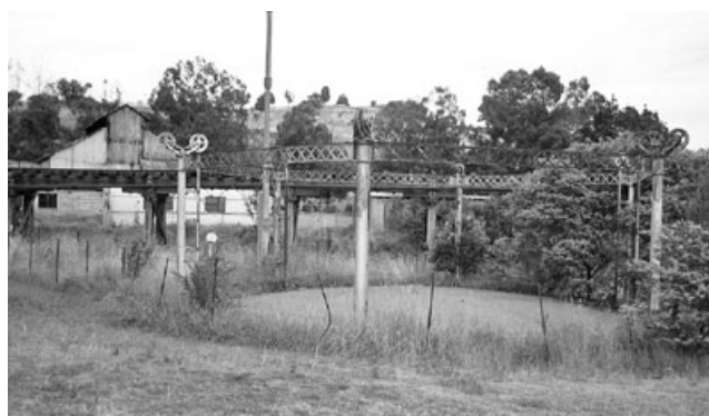
Remediation of the former Yass gasworks commenced this year
