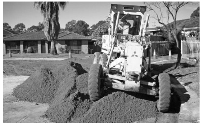
Trialling recycled road base at Fairfield
