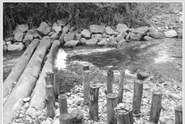
A log sill helps slow the flow of water and prevent erosion of the riverbed
