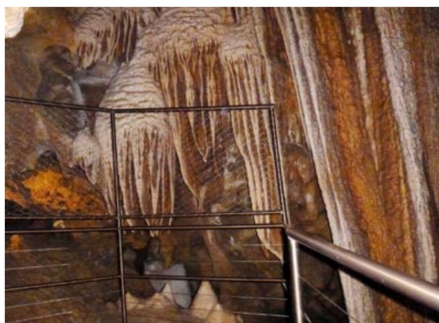
New stainless steel railings in the Jenolan Caves.
