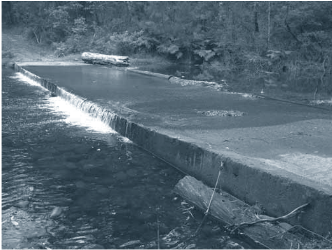
Road crossing blocking fish passage
