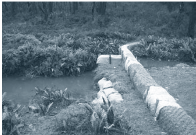
Swamp rehydration works at Marmion Swamp, North Katoomba
