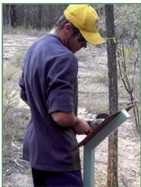
Installing the interpretive signs
