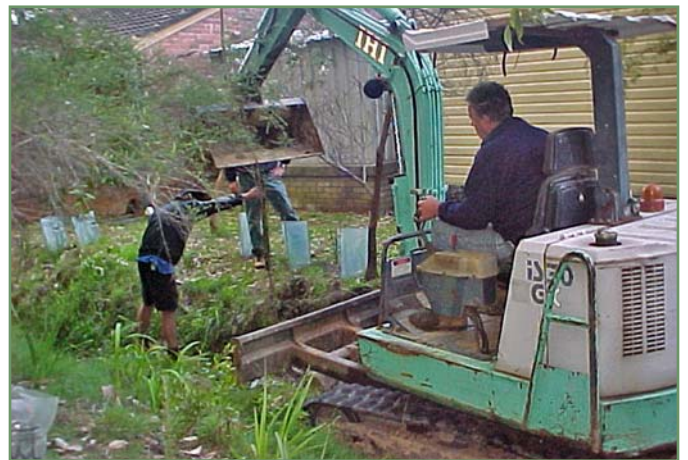
Clearing and revegetation work in progress
