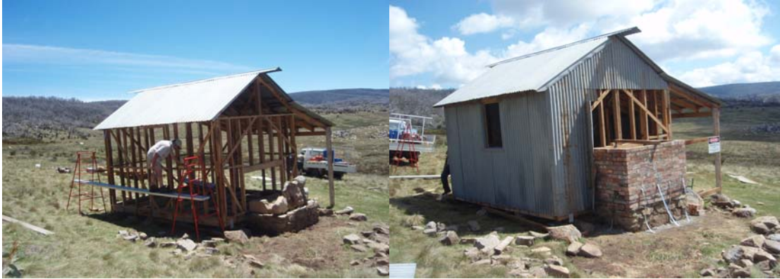
Brooks Hut rebuild. Photos: Megan Bowden DECCW
