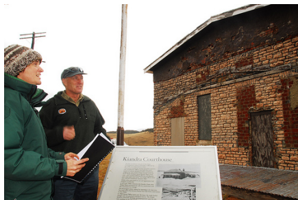
Kiandra courthouse – removal of cement render on exterior walls. Photos: Jennifer Hewitson DECCW
