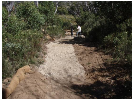
Thredbo Valley Track March 2009 stone pitched causeway and local granite surface material. Photos: DECCW
