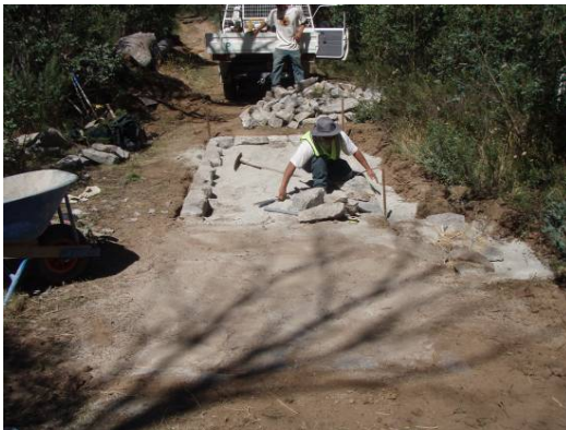
Thredbo Valley Track March 2009 stone pitched causeway and local granite surface material. Photos: DECCW
