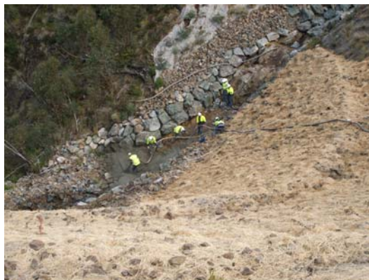
Shotcrete work on the drainage line at Tumut Ponds hairpin site Photo: DECCW
