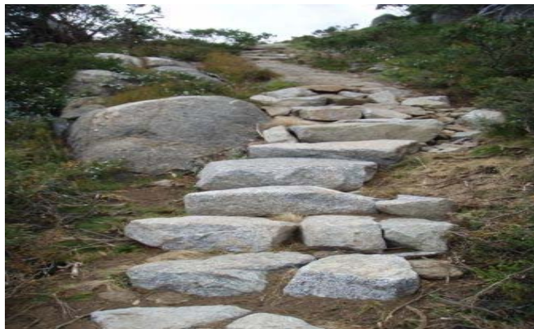
Stillwell walking track construction. Photo: DECCW
