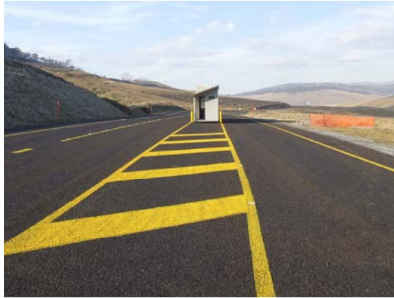
New Mt Selwyn Visitor Entry Station and road works. Photo: DECCW
