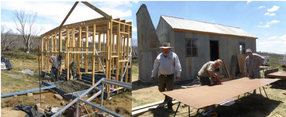
OKeefe's Hut rebuild. Photos: Megan Bowden DECCW
