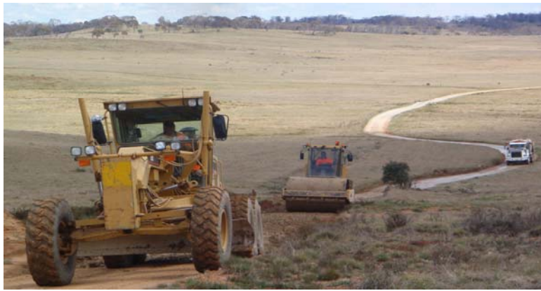
Port Phillip Trail – grading and gravel sheeting. Photo: DECCW
