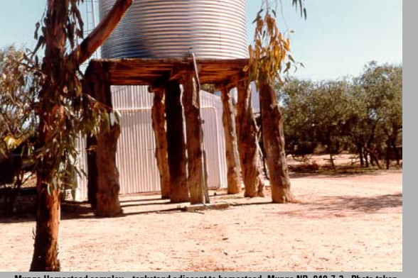
Mungo Homestead complex – tankstand adjacent to homestead, Mungo NP, 049-7-3. Photo taken 30-4-1985 by E Rich.
