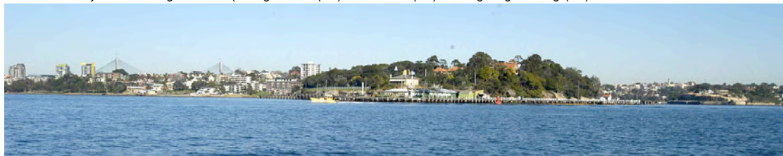
Figure 3.40 A more distant view of the island from the east. From this distance the northern built elements, particularly the Water Police Station (47) retain some visual dominance but the vegetated form continues to dominate the view. The Harbour Master's Residence and adjacent cottages are virtually hidden by vegetation.
