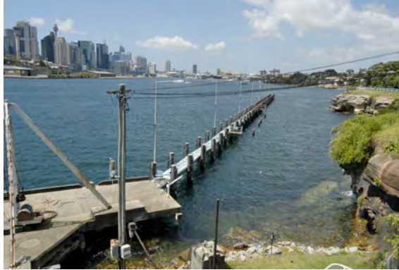
Figure 3.46 The view from the roof of the Port Emergency Services Building (45) looking south along the shoreline of the island towards the city and Darling Harbour. The flat roof of the building provides a large viewing platform with uninterrupted panoramic views.
