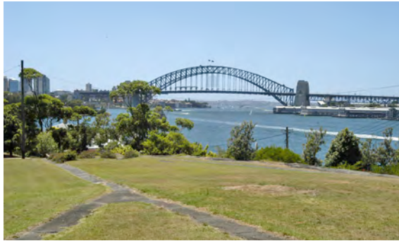
Figure 3.50 The view from the front verandah of the Harbour Master's residence (39) showing the orientation of the dwelling directly down the harbour (but slightly obliquely to the bridge which was constructed later). The importance of the location of the residence, its direct views and its prominence were part of the initial design of the facilities on the island by the SHT.
