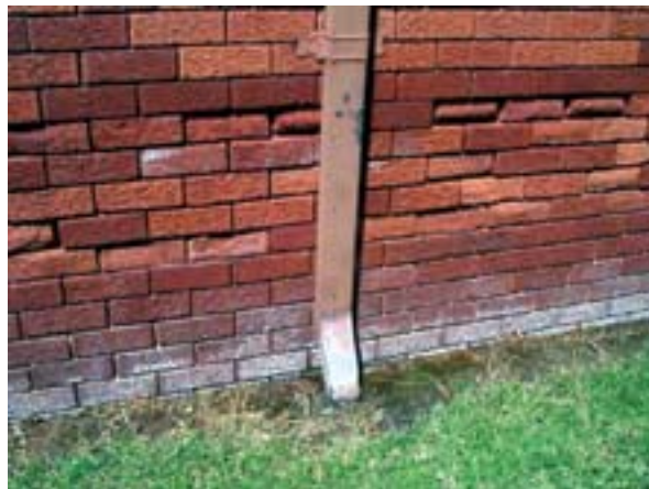
Rusted down pipe allowing rainwater to mobilise salts in the soil. - Photo: DIPNR
