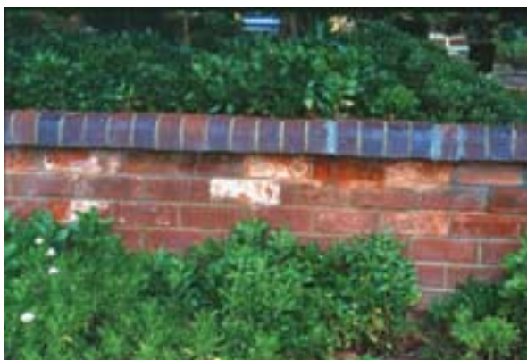
Non exposure grade bricks used in a garden wall Photo: NSW Agriculture
