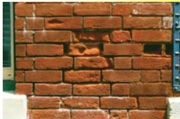
Bricks showing signs of salt and water damage Photo: NSW Agriculture
