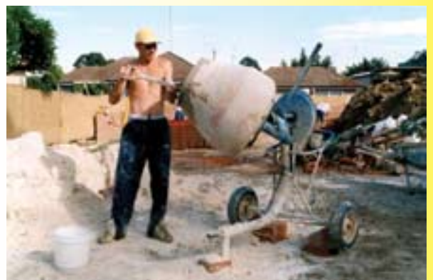
Concrete being mixed on site - Photo:DIPNR
