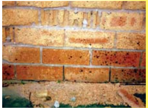
Brick work showing the effects of fretting and the accumulation of brick 'grains' at the base of the wall Photo: DIPNR
