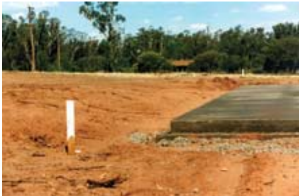
Typical slab on ground construction. - Photo: DIPNR
