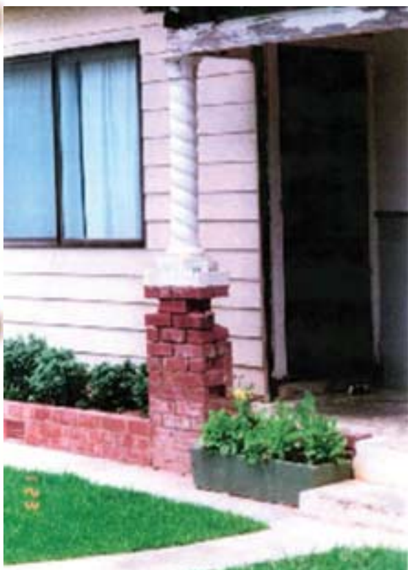
Verandah post showing signs of salt and water damage
