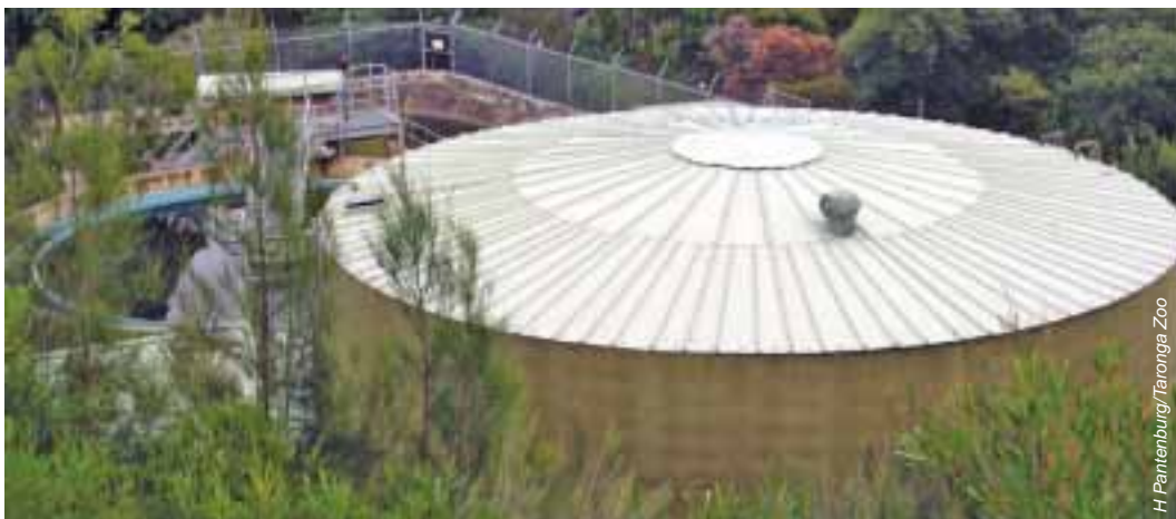
Taronga Zoo stormwater and wastewater treatment plant
