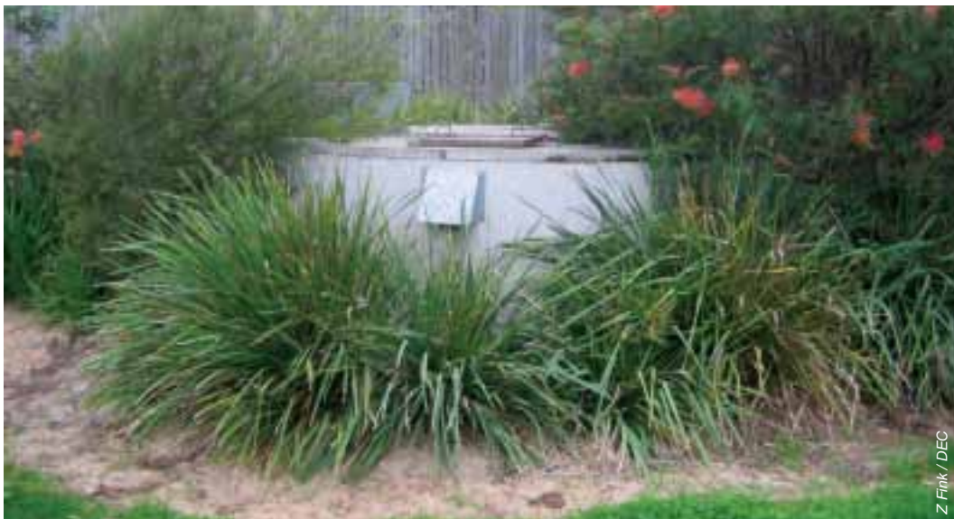
Irrigation storage tank, Powells Creek Park
