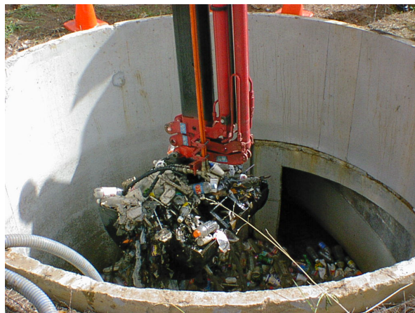
Gross pollutant traps like the one above installed through the Stormwater Trust Grants Program, will stop over 3600 tonnes of pollution entering NSW waterways each year.
