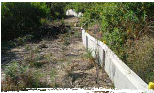
Figure 20: A sediment fence at a remnant in Wassel Street, Randwick, actively prevents encroachment of certain weed species
