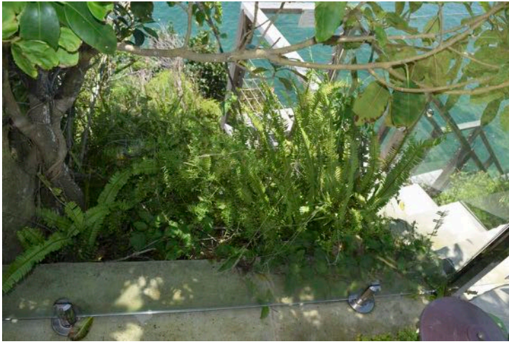
Weeds to be trimmed beside stairs on north side.
