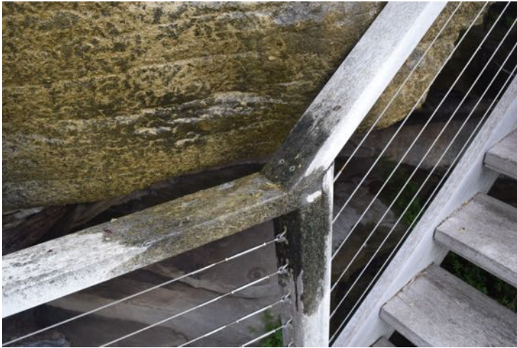
Water dripping onto hand rail.
