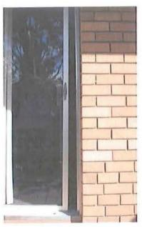
Photograph showing the dislocation of a door-frame from its adjacent brick-work — caused by the tree roots lifting the foundations of the house.
