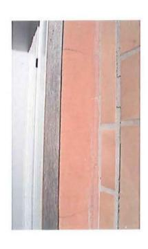
Photograph showing the effect on the alignment of a door in relation to its frame caused by the tree roots lifting the foundations of the house
