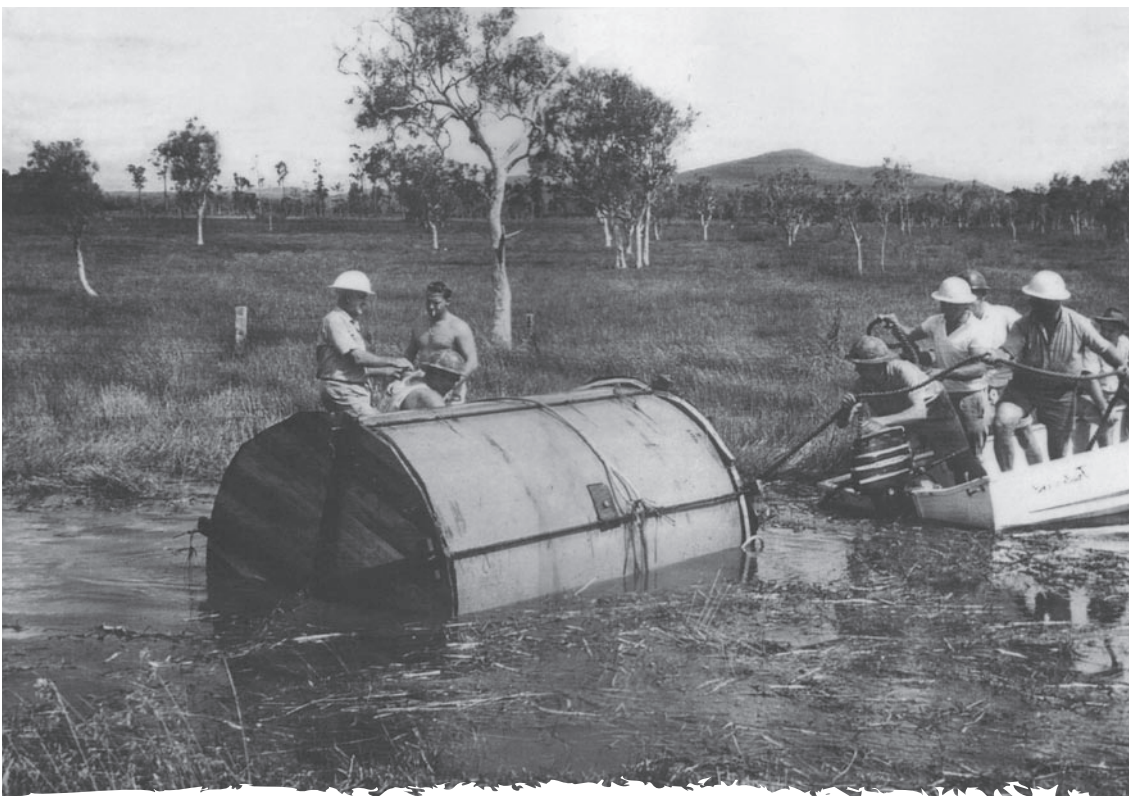
Pipe being floated over a wetland during the 1966 construction of the Taloumbi Radial drains, that now drain into Lake Wooloweyah (Clarence Valley Council)
