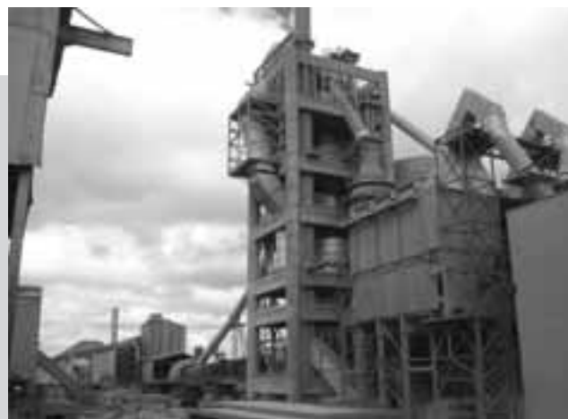
This kiln at the Blue Circle cement works at Berrima is being used to trial alternative fuels.
