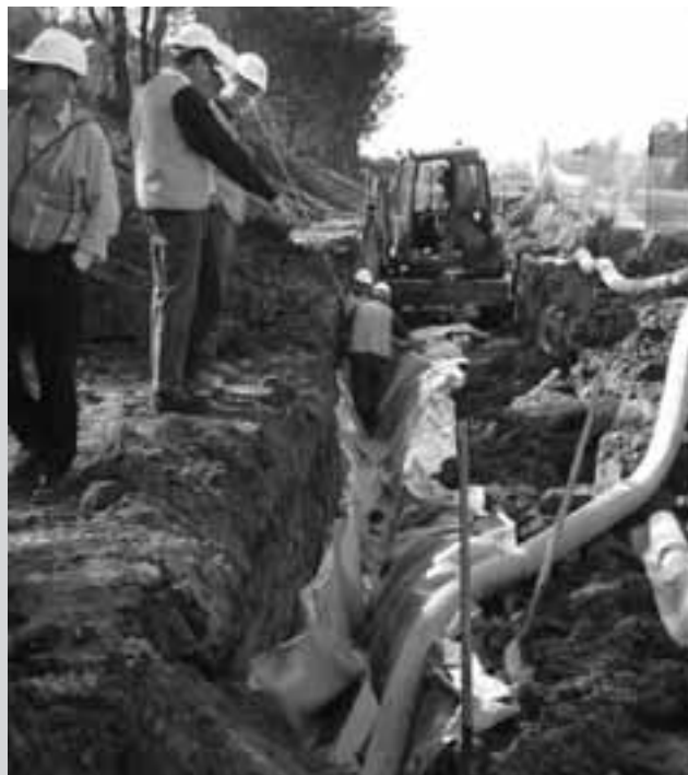
Installation of the leachate collection system following construction of the in-ground leachate cut-off wall.
