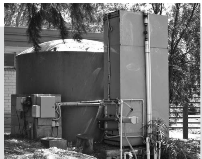
Lane Cove River Tourist Park's grey water recycling system contributed to water savings of one megalitre in 2008.
