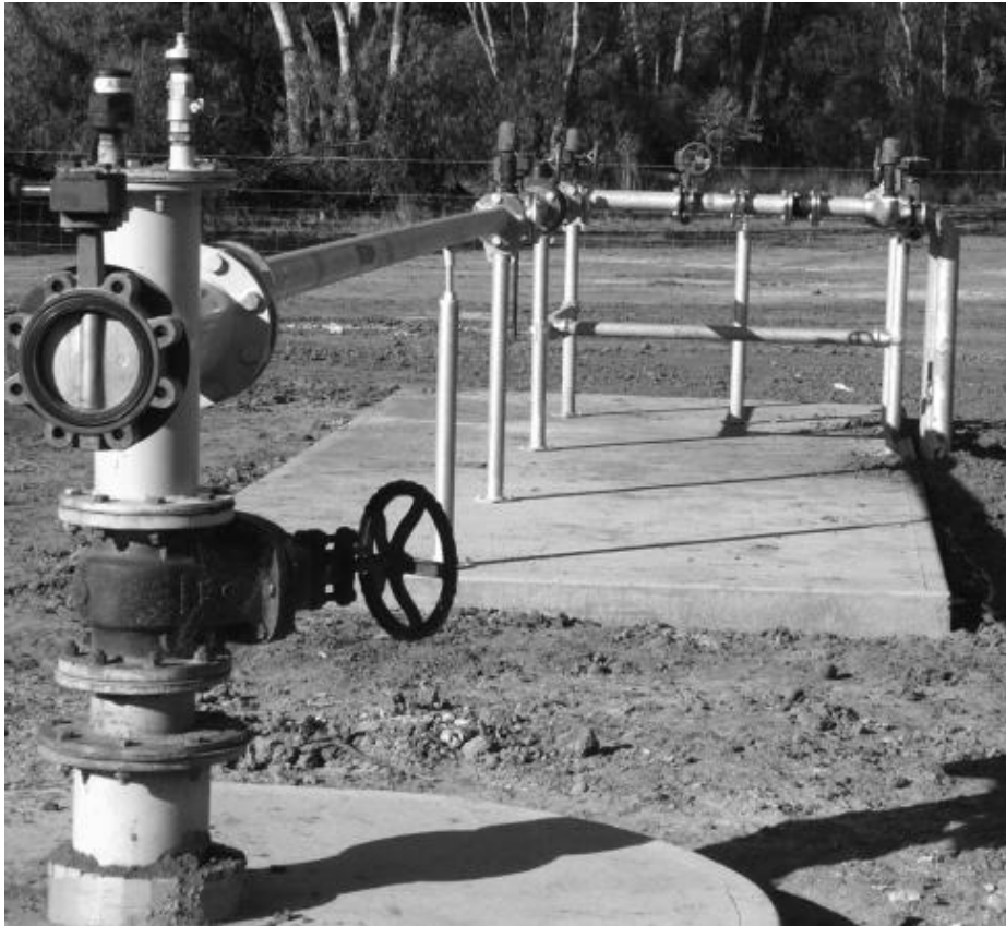
Bore after capping and piping.
