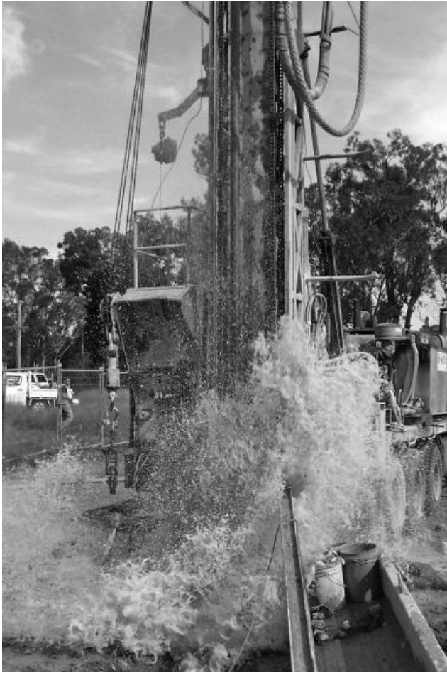
Airlifting groundwater to clean a hole following a change of rods during bore drilling.
