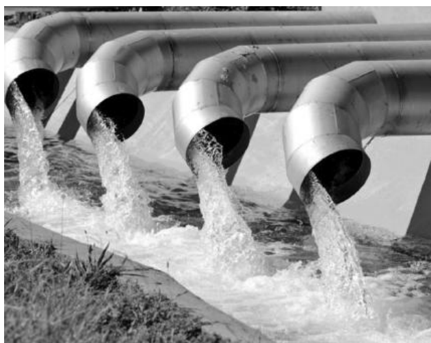
Water from the recycled water plant at St Marys is piped to Penrith, where it is released into Boundary Creek before entering the Hawkesbury–Nepean River.
