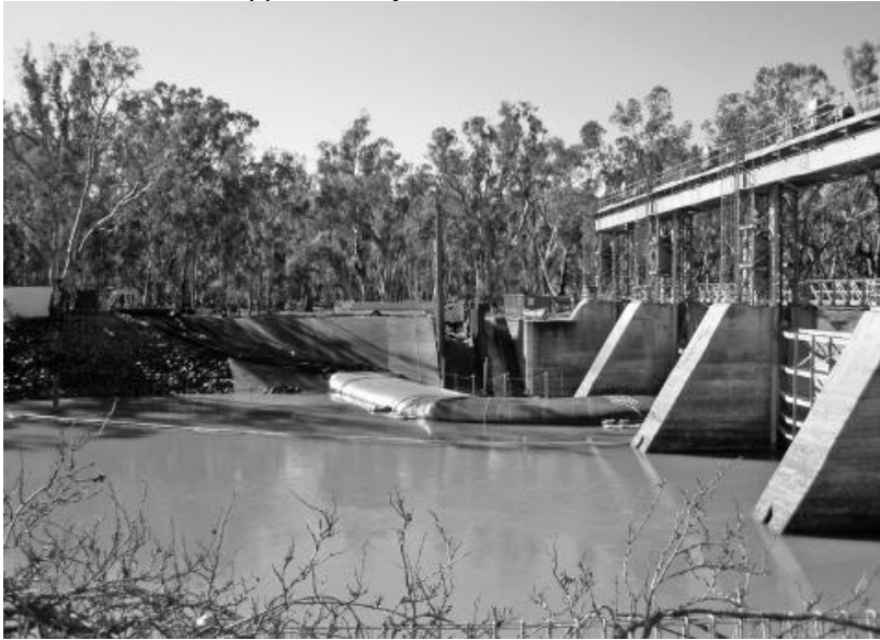
Steven's weir fishway under construction, showing the downstream entrance.
