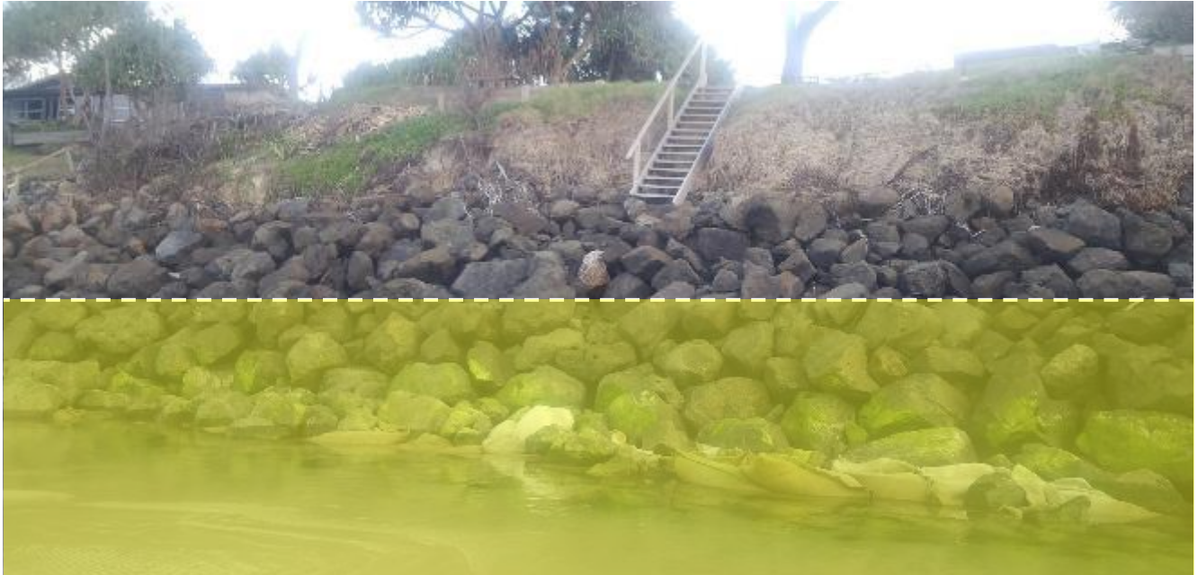
Figure 7 Toe and adjacent wall to southward exposed during erosion in 2013 (ICM photo). Dotted white line shows approx. present sand level (about +1.8m AHD). Sand bags placed along original toe are exposed.
