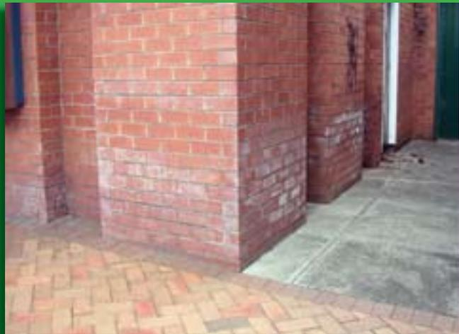
**Fig. 3** White staining indicating the growth of salt crystals on the surface of brickwork. Photo: A. Collings
