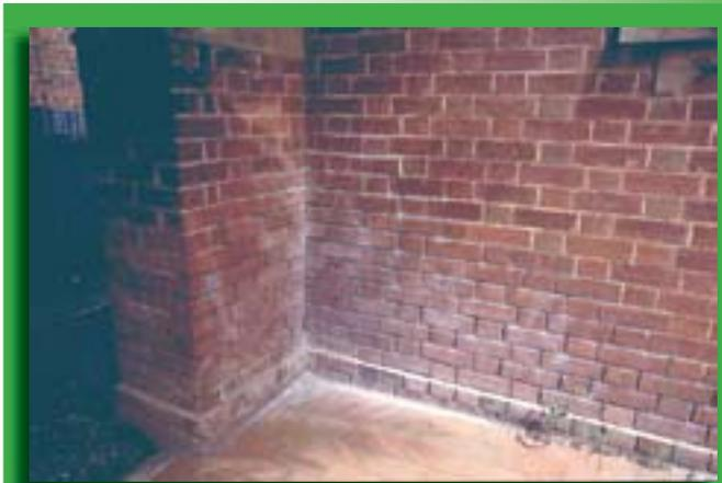
**Fig. 6 Severe breakdown and loss of mortar with accumulation of powdered mortar around the base of the wall. Photo: A Collings**
