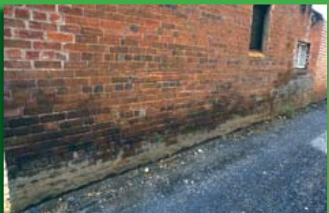
**Fig. 4** "Tide mark" caused by rising damp. Photo: A. Collings
