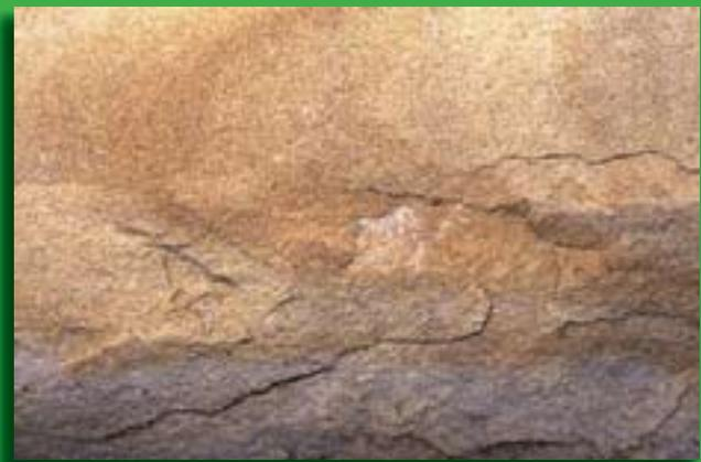
**Fig. 12** White staining and flaking of the sandstone surface caused by the growth of salt crystals and rising damp.
