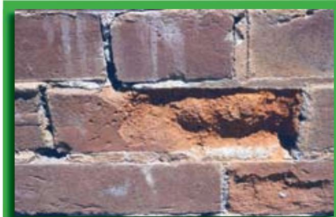
**Fig. 5 Mechanical breakdown of brickwork caused by rising damp and the growth of salt crystals. Photo: A. Collings**
