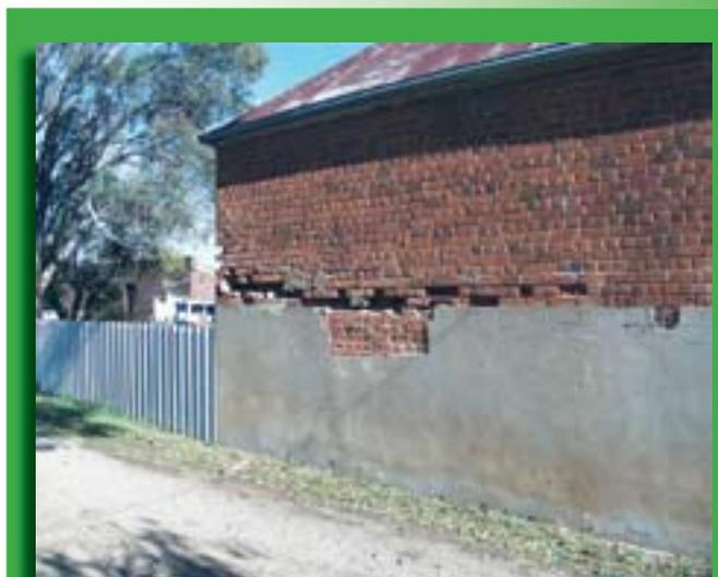
**Fig. 7 Cement render has aggravated rising damp leading to damaged brickwork further up a wall. Photo: DLWC Library Cowra**
