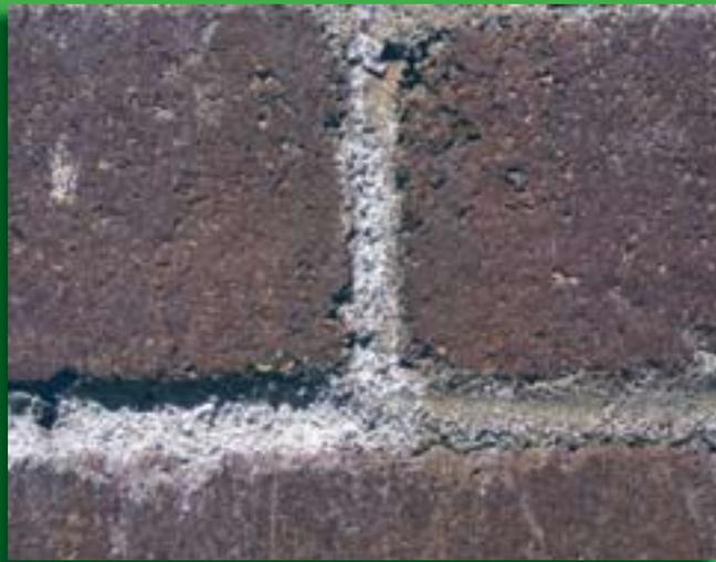
**Fig. 2** Early signs of mortar break down caused by growing salt crystals and rising damp. Photo: A. Collings
