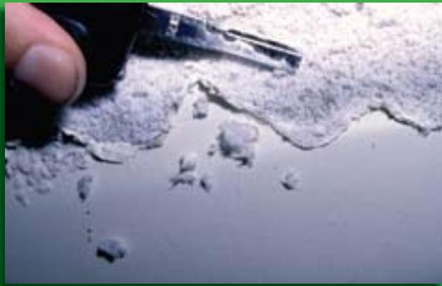
**Fig. 8** Growth of salt crystals through blistered paintwork. Photo: A. Collings
