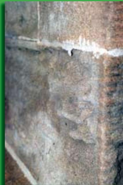
**Fig. 13** White staining and loss of the surface of sandstone caused by rising damp and salt.
