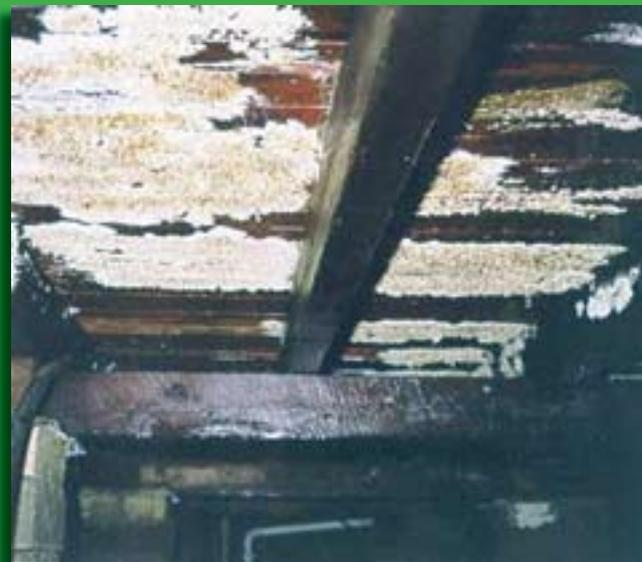
**Fig. 9** A consistently high watertable around house foundations has led to rotting of timber floorboards and joists. Photo: DLWC Library Cowra
