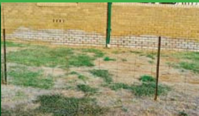
**Fig. 22** Raised saline groundwater has led to the partial death of this lawn. Salts have also built up on the surface of brickwork below the damp course. Photo: DLWC Library Cowra
