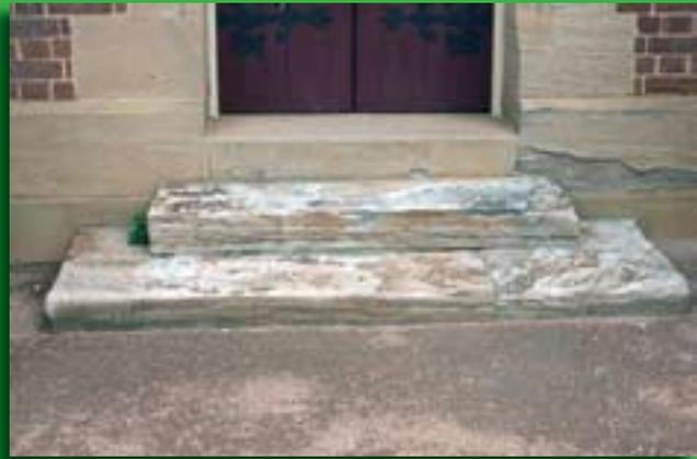
**Fig. 11** White staining and erosion of the tread of a sandstone step caused by salt.
