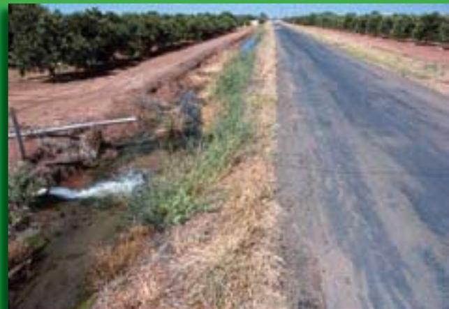
**Fig. 18** Rutting and breaking up of road surface due to saturation of the underlying soil and the roadbase. Photo: A. Collings
