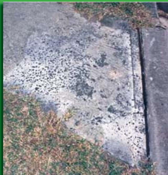
**Fig. 16** Sulphate attack of the cement component in a concrete footpath has exposed the aggregates. Photo: A. Collings
