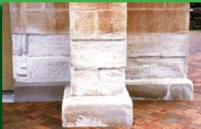
**Fig. 10** Bleaching of sandstone caused by salt and rising damp Photo: A. Collings
