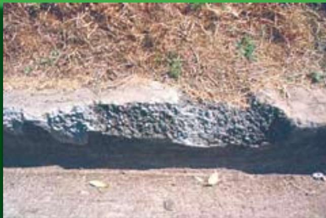
**Fig. 15** Sulphate attack of the cement component in concrete kerb and guttering has exposed the aggregates. Photo: A. Collings
