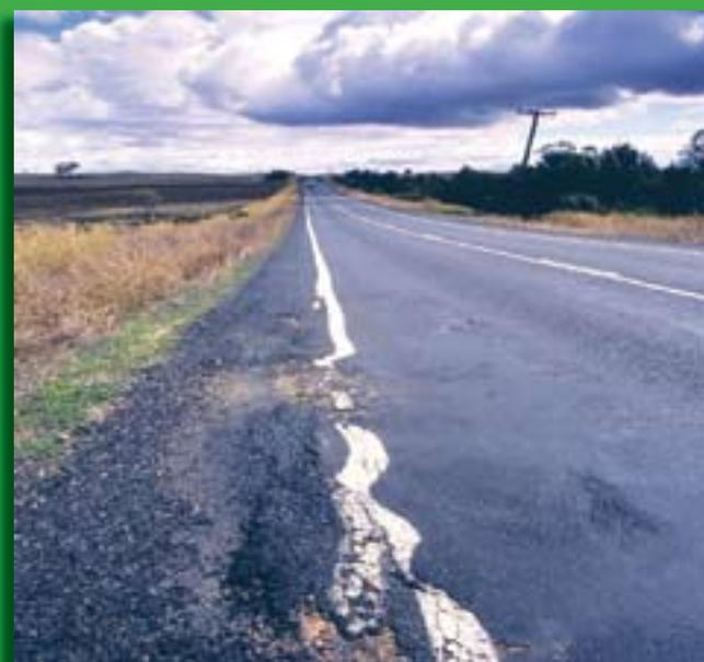
**Fig. 19** Disruption of natural drainage lines has caused a build-up of ground water next to the road. This has led to rutting and potholing of the road surface. Photo: A. Collings
