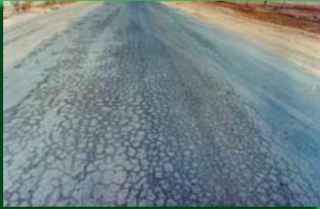
**Fig. 20** Saturation and salinisation of the road base is leading to premature breakdown of the road surface. Photo: DLWC Library Cowra
