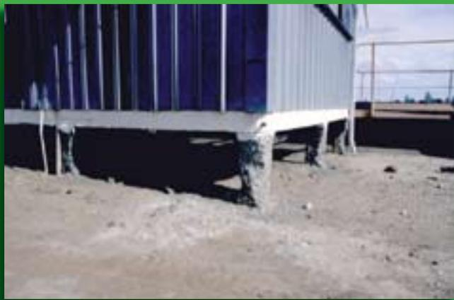
**Fig. 14** Breakdown of concrete piers caused by salt induced corrosion of the steel reinforcing in the concrete. Photo: A. Collings
