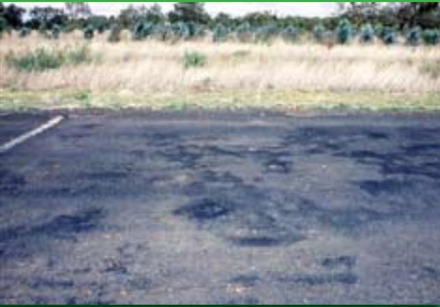
**Fig. 21** Water and salt build-up between the asphalt surface and the road base has led to potholing and delamination of the road surface. Photo: A. Collings
