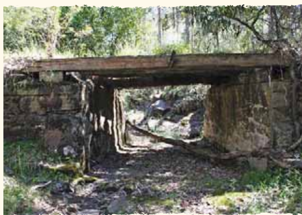
This historic sandstone bridge over Woodhouse Creek on the Beulah biobank site was constructed in the 1830s. It is the only one of its type in Australia to retain a full set of stringer girders. Photo: OEH.
