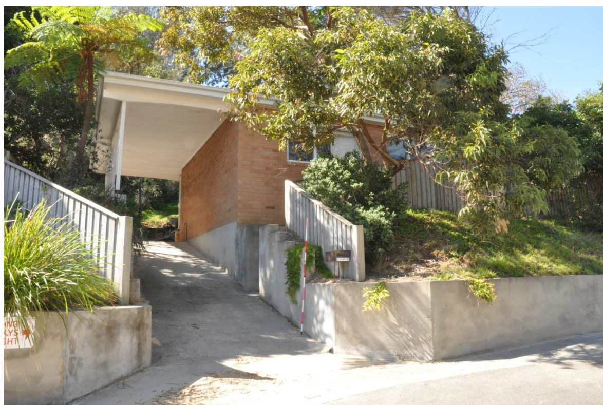
Figure 3.3 Image showing the elevated (filled) platform on which 33 Cliff Street has been constructed. (Source: GML 2015)
