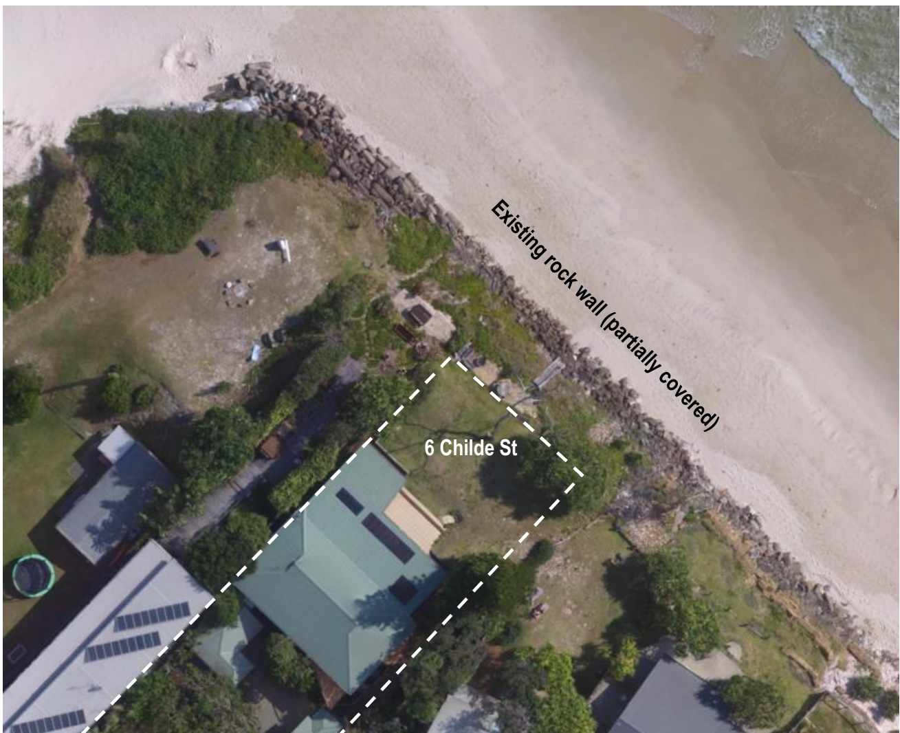
Figure 1 High definition aerial image of 6 Childe Street (ICM 13/10/16)
