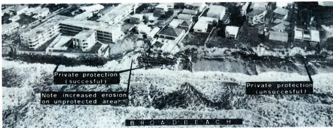
Figure 2: End effects and potential flanking of seawalls, Gold Coast 1967 (Source: Delft, 1970)
