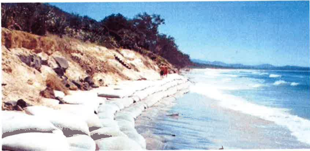
Figure 1: Traversing geotextile container walls, Belongil January 2002 (photo: James Carley, WRL)
