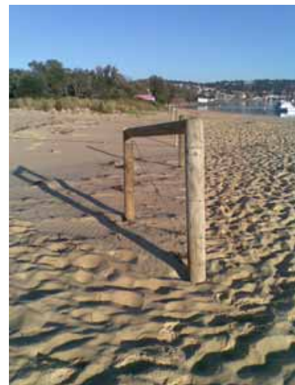
Figure 3: Fencing was extended at the northern end for dune regeneration and rebuilding without pedestrian traffic.
