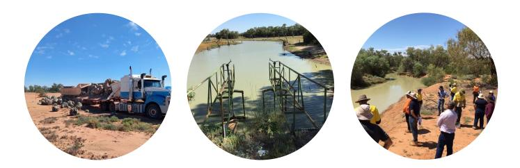
The new structures at Boera and Homestead dams will enable more water to flow to the Darling River when downstream needs are a priority and provide for ongoing watering of important habitats on Toorale when needed. Fishways will increase connectivity and support healthier fish populations in the Warrego and Darling rivers.
