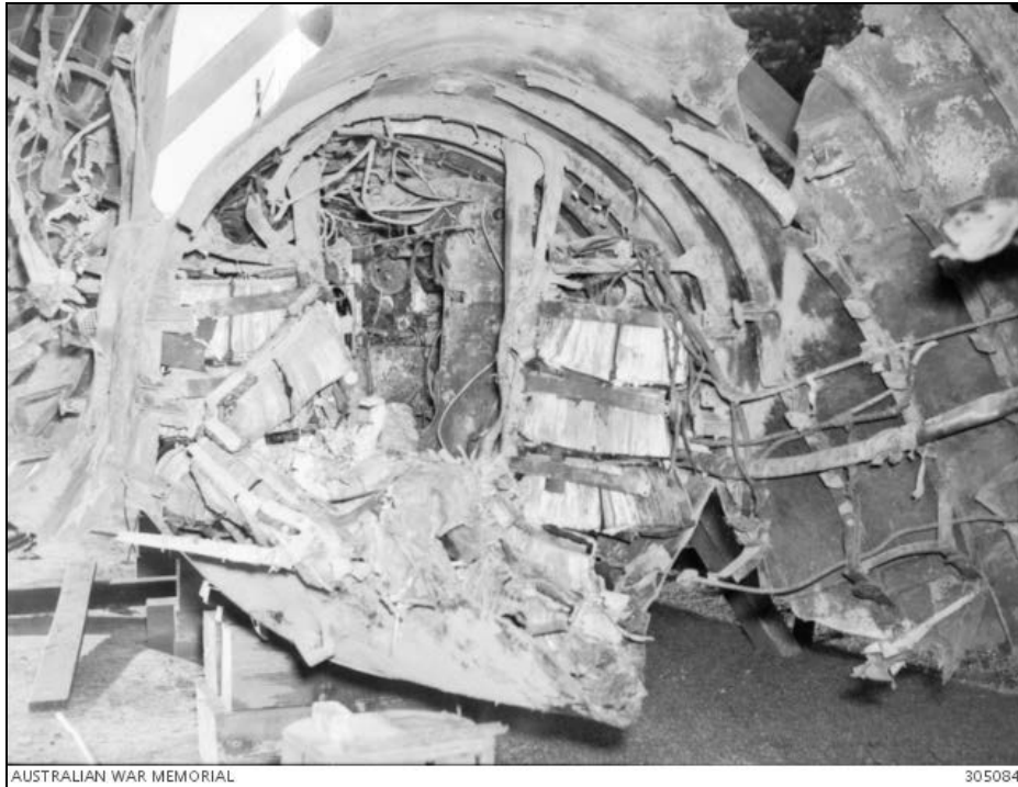
Figure 16: View of detonation area in forward battery compartment of Ha-14 looking aft to control room (Image: AWM 305084, AWM Collection).
