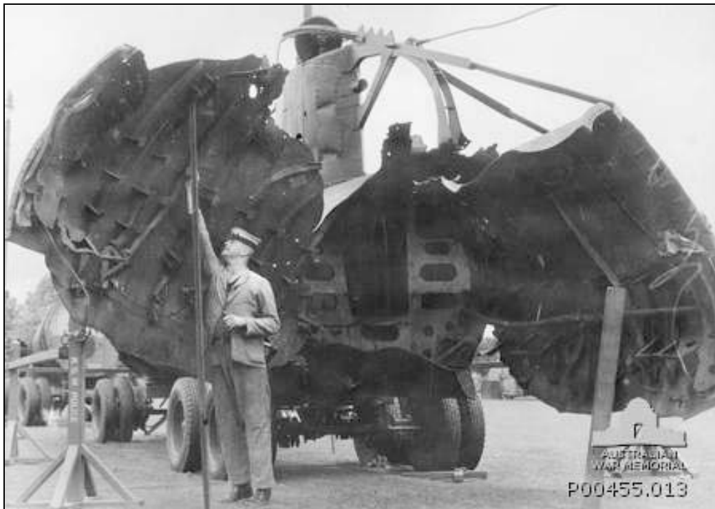
Figure 11: Picture showing exploded hull of the Ha-14 Midget Submarine after being cleaned up for exhibition (Image: Herald Newspaper 1942 - AWM P00455.013).
