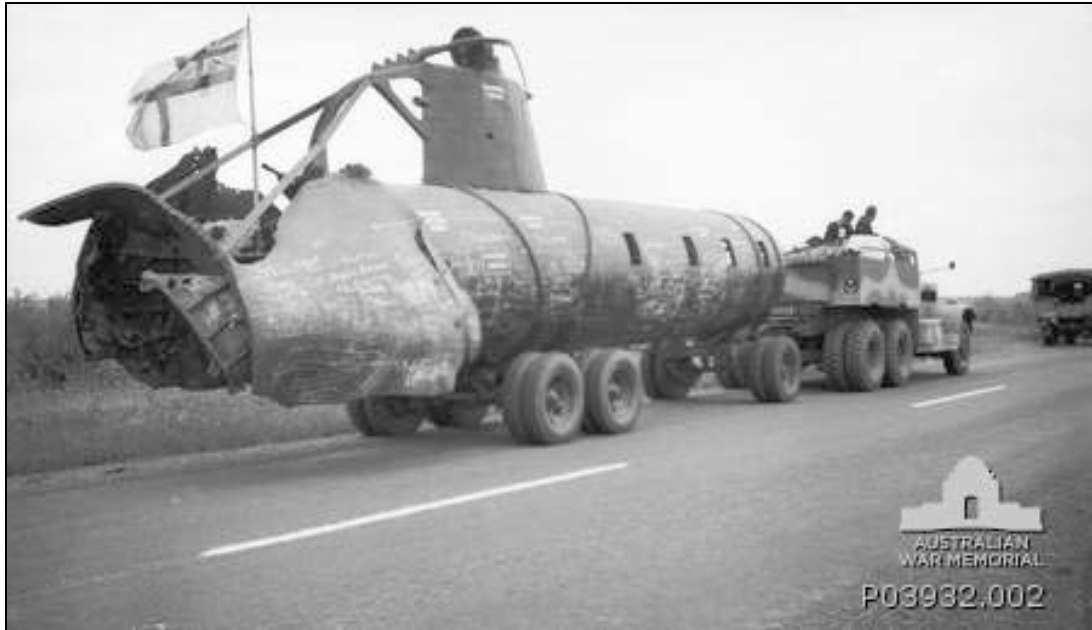
Figure 12: Midget submarine on trailer on touring exhibition showing mangled forward end of the submarine minus torpedo and engine rooms (Image: Goggs 1942 - AWM P03932.002).
