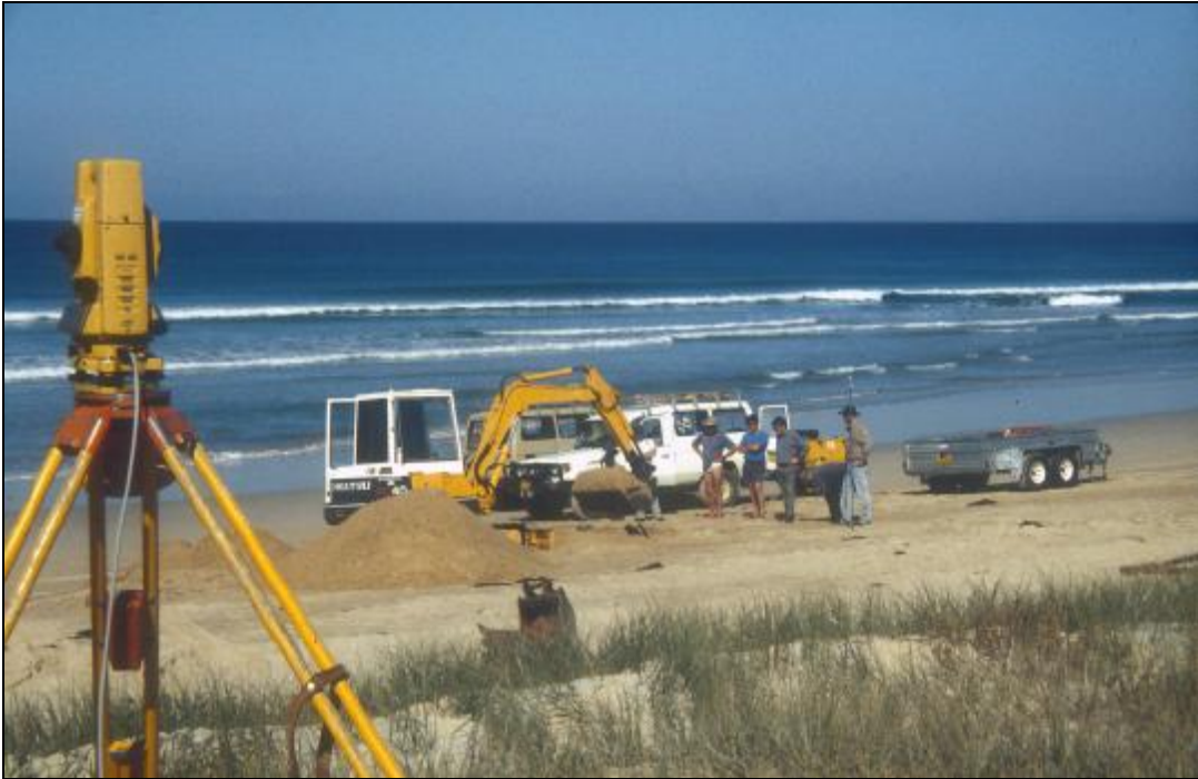
Figure 8: Position fixing was achieved by a combination of differential GPS and a Topcon Total Station theodolite.
