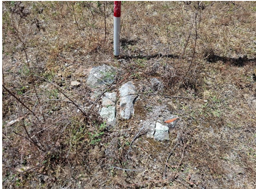
Figure 14: Small outcrop of weathered meta-sedimentary bedrock showing jointing/fissility cracks. Observation confirms a shallow and variable soil cover over bedrock in the area of proposed works.
