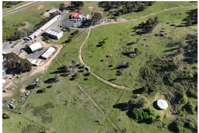
Figure 13: View to the proposed facility location
