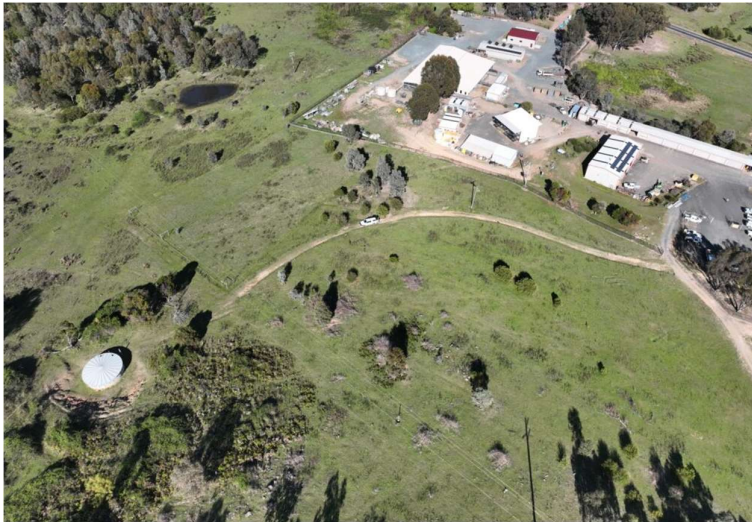
Figure 2: Aerial view to the proposed facility and existing access track location
