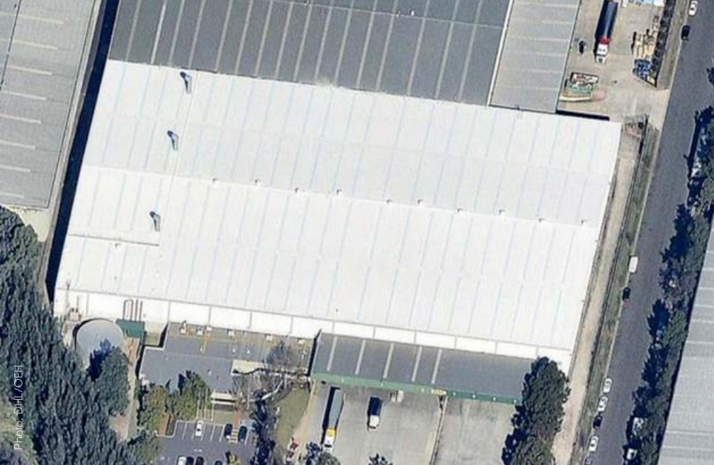
Warehouse A roof with solar reflective coating
