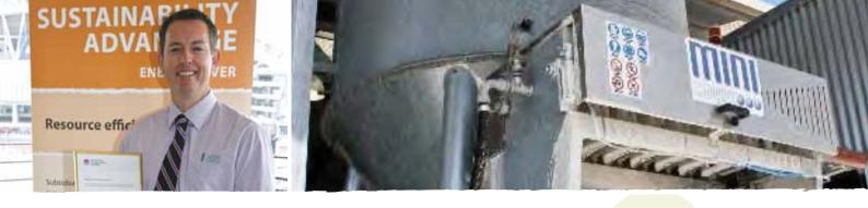
▶ Edstein exceeded expectations. Initially, the firm cut its water use by 97 per cent – from 24.5 megalitres per year to 0.6 megalitres. Now, Edstein does not draw any water from the main water supply. Not a drop. This remarkable achievement is possible by harvesting rainwater from the large factory roof into a 250,000-litre tank – the firm's new water source.
