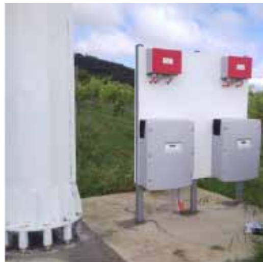
Figure 6.1: Two SMA 5 kW inverters and controllers (Photo: Enhar)
