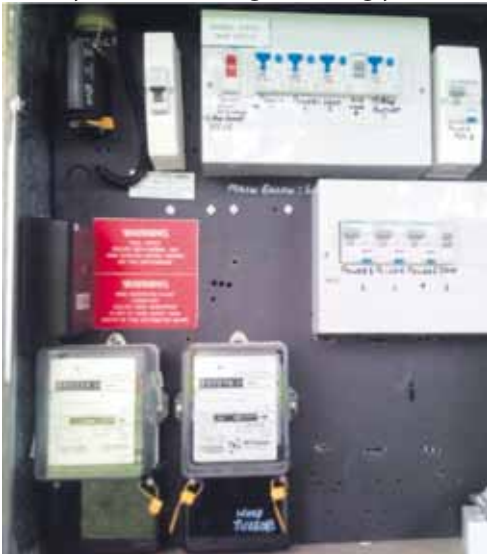
Figure 5.3: Photograph of gross meter arrangement [courtesy of Rewind Energy]
