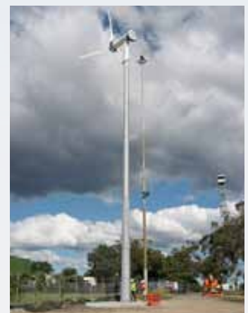
Hornsby - 15kW turbine for rural fire station
