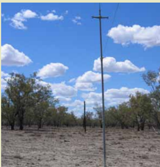
Telegraph line of single-strand wire strung between wood and steel poles, Culgoa National Park. Photo: Stirling Smith/DECCW, 2006.
