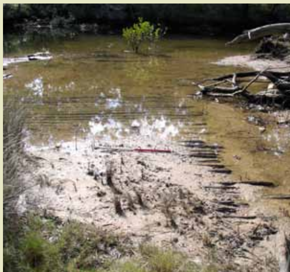
Cut timber ('corduroy') crossing at Saltwater Creek, Yuraygir National Park. Photo: Dan Tuck/DECCW, 2006.
