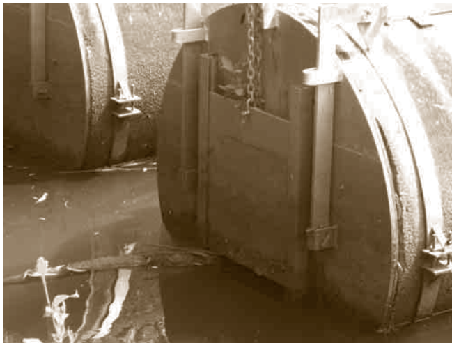
Open floodgate to allow fish passage and water flow
