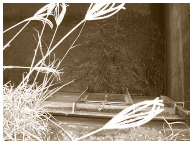
Open floodgate allowing water exchange and fish passage
