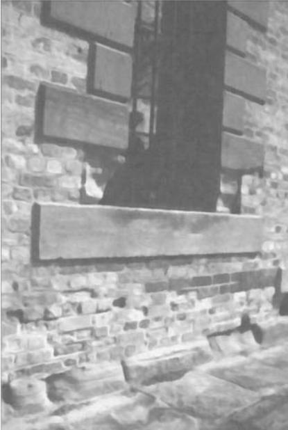
*Rising damp in brick and stone masonry. Note how the worst decay is at the base of the window opening. This is where most evaporation takes place and hence most decay due to salt attack.*
