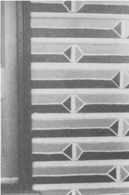
*The example of painting onto decorative weatherboards seeks to imitate rusticated stone. It can be observed from the surface patterns that the shading was achieved by using different paints of unequal properties.*
