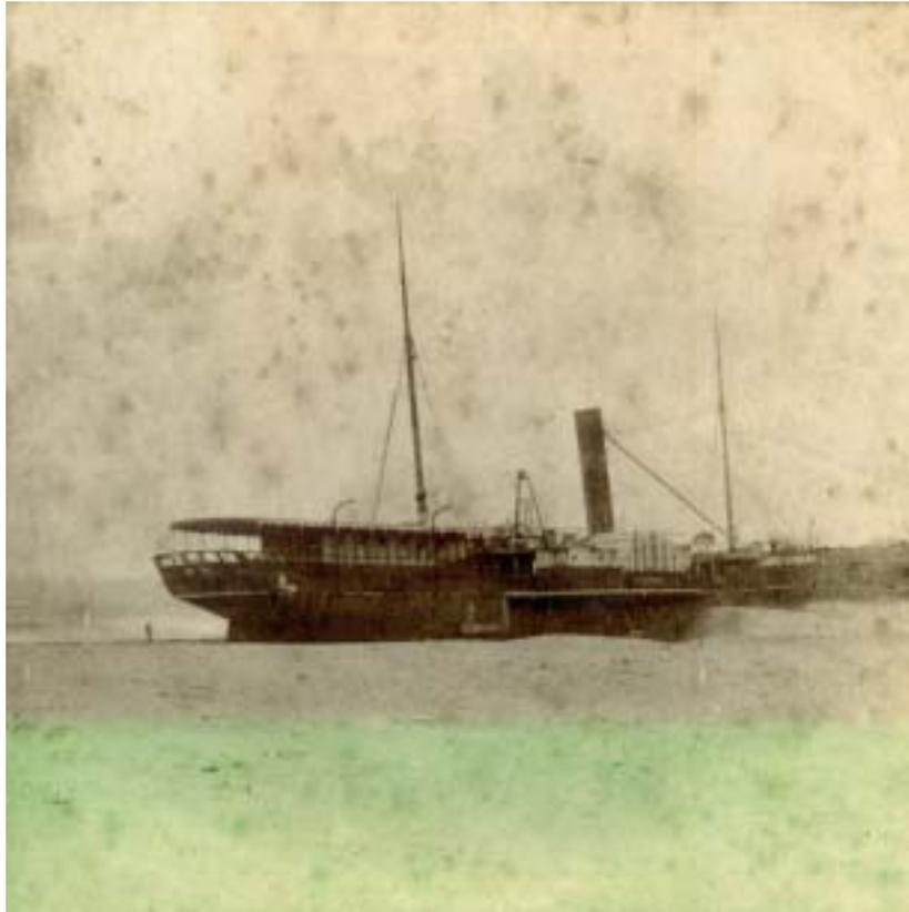
**Figure 7** *The Collaroy after some time ashore. Notice the build up of sandbanks around the beached hull. Probably taken at time of 1884 recovery operations due to the form work evident around the hull and boarding ladder onto sponsons. Photo courtesy: Macleay Museum, University of Sydney.*
