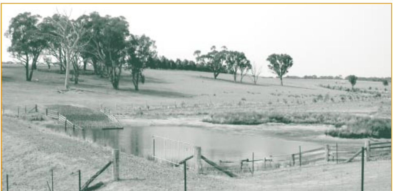
Figure 3.6 Provide a gravelled stock ramp into fenced off dams
